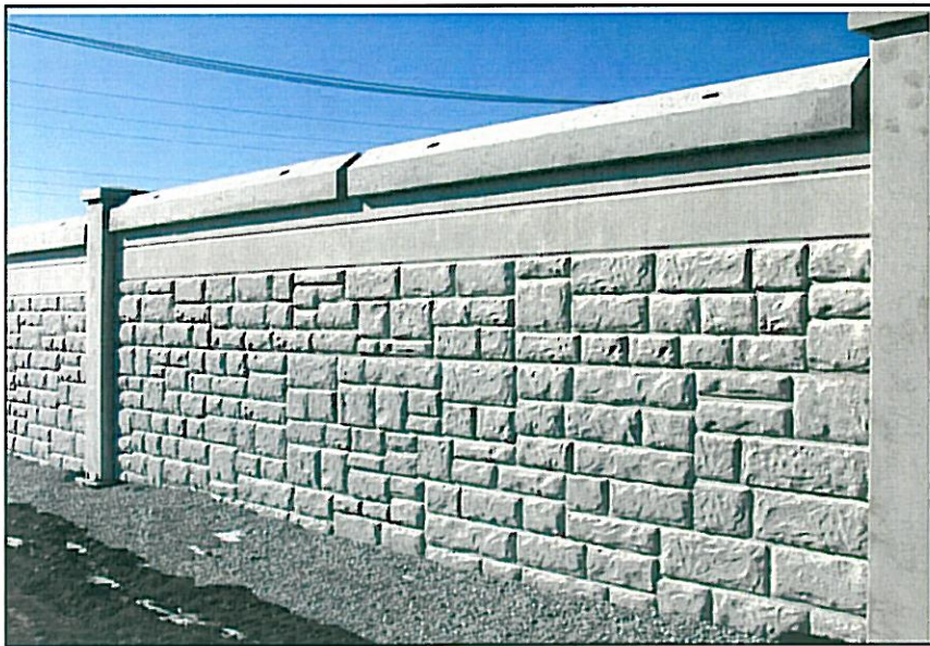
Electrical Substation, St. Louis, MO
